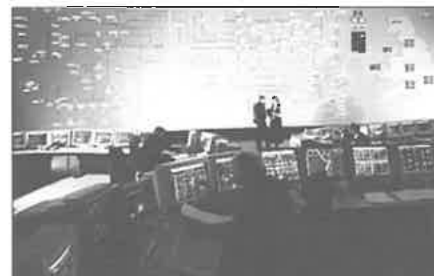
Slika 1 – Kontrolni centar "National Grid Company" u Reddingu, UK
